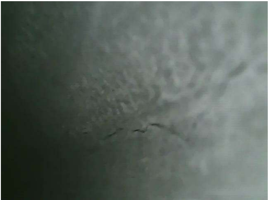
Photograph 7 - Second crack to lower nib
