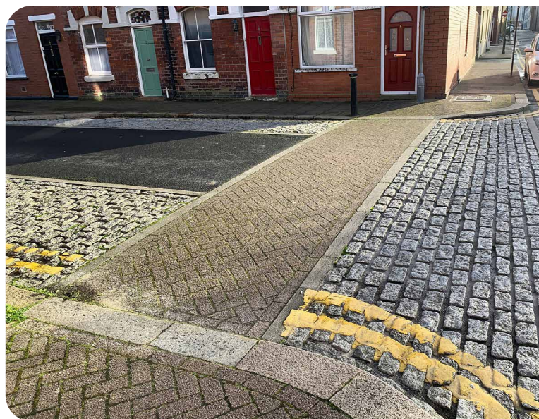
Boundary Treatment on Keith Street
